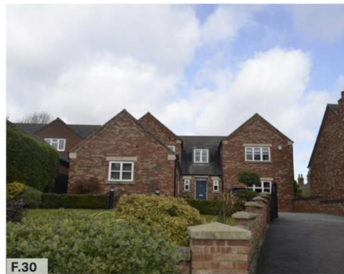
Figure 30: Example of on-plot garage parking, Whissendine.
