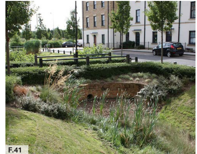
Figure 41: Example of swales check dam integrated with a crossing point elsewhere in uk.
