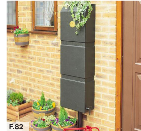
F.82 Figure 82: Example of a gravity fed rainwater system for flushing a downstairs toilet or for irrigation.
