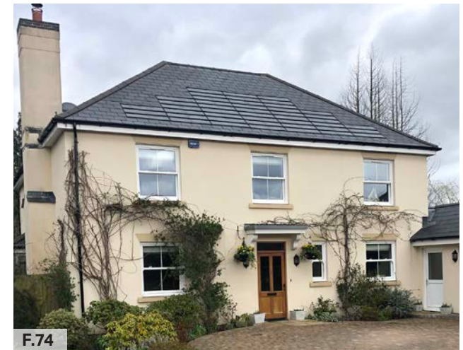
Figure 74: Use of shingle-like solar panels on a slate roof, with the design and colour of the solar panels matching those of the adjacent slate tiles.
