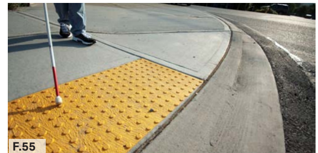
Figure 55: Example of tactile paving to facilitate movement for people with visual impairment.
