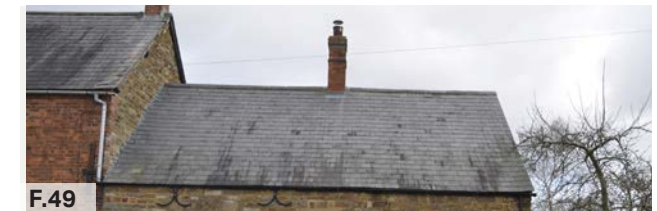
Figure 49: Local examples of roof materials that could be used in new development, e.g. grey slate and clay pantiles.
