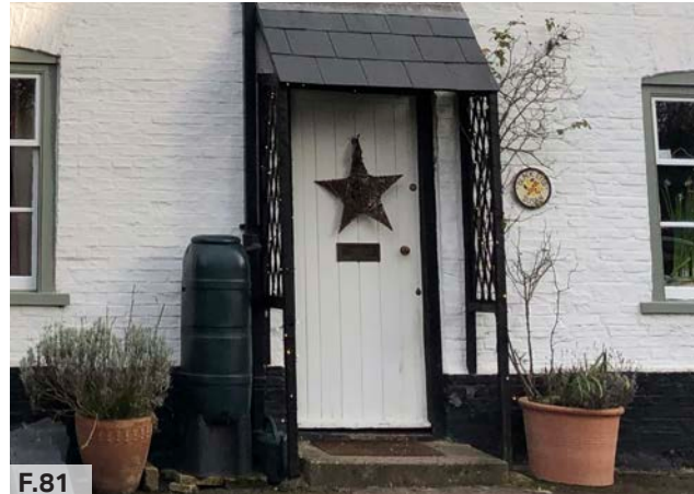
F.81 Figure 81: Examples of water butts used for rainwater harvesting in Reach, Cambridgeshire.
