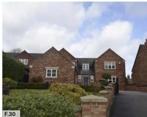
Figure 30: Example of on-plot garage parking, Whissendine.
